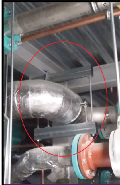
We fix to steelwork and purlins
