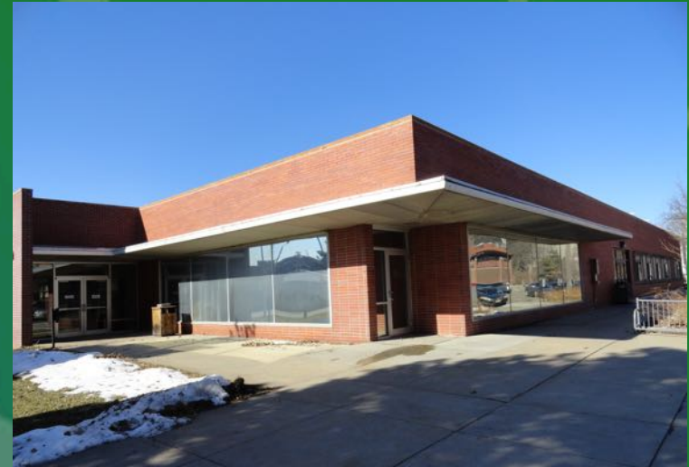
501 Building – The first building audited by the students
