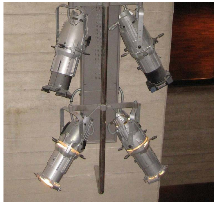
National Theatre: Conversion of ETC Source 4 projectors to use CDM-T Elite 70W lamps.
