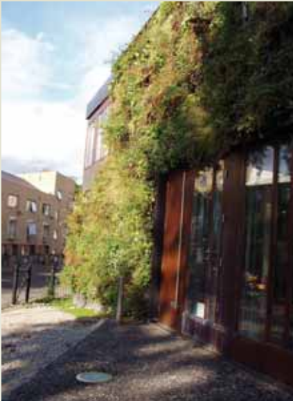
Figure 4: 'Green' wall at a community centre in Paradise Park, Islington
