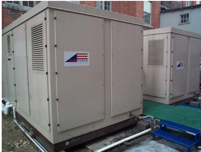
Figure 1 UTC PC25C PAFC - The only commercially available fuel cell
