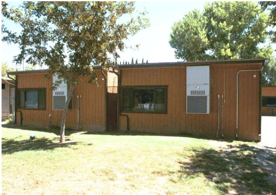
Figure 1 - School Site Test Rooms – Rear View Looking East
