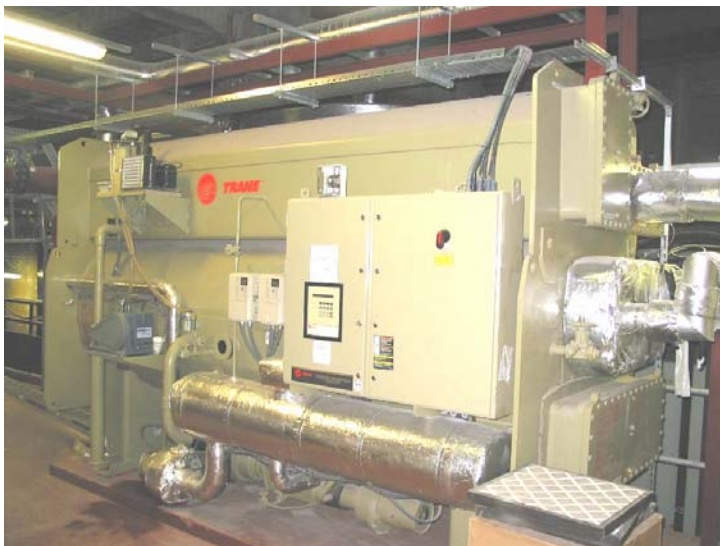
600kW absorption chiller
