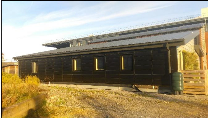
Figure 14 Solar Collectors on the Active Classroom (south facing)
