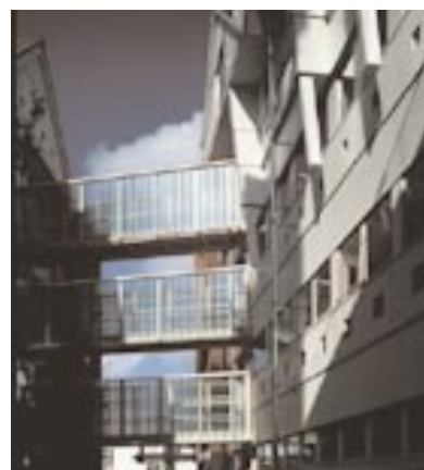
Figure 4 Stepped white façades and opening windows on courtyard elevations of electrical laboratories
