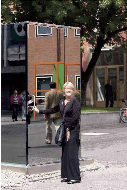
The all new Public Convenience (From the outside)
