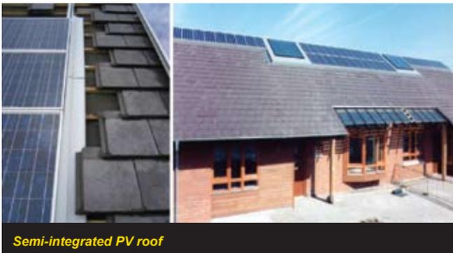
Semi-integrated PV roof
