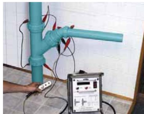
Fusion controllers have also improved to make installation as simple as possible. The CPV Zurn control box can weld several joints simultaneously, triggered remotely from a hand-held switch, if required. A USB memory stick connection offers a very
