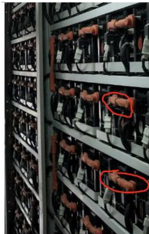
Dust over cooling pipe and IGBT devices
