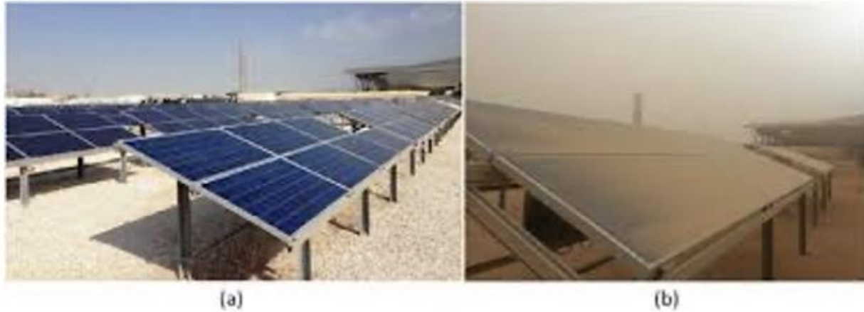
Dust on PV module in comparison
