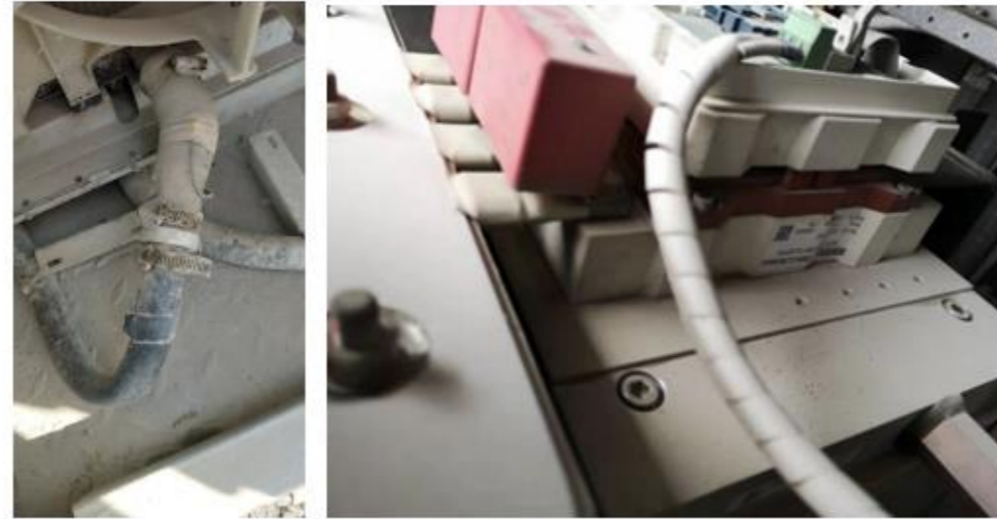
Dust over cooling pipe and IGBT devices
