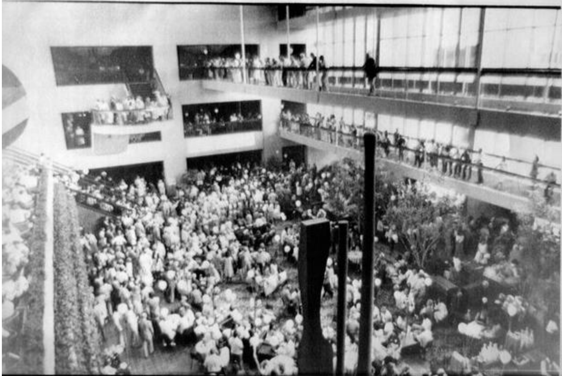
(PHILADELPHIA, CAMDEN, WILMINGTON OUT--MO--MO--COPYRIGHT: DORIS NEWMAN) (FX9--July 20) HYATT TEA DANCE--Spectators on overhead walkways watch people below during a tea dance at the Kansas City Hyatt Regency Hotel on June 19, 1981. One month later, the uppermost walkway, extreme top center, fell on the lower walkway sending people and debris from both walkways spilling onto the crowded dance floor below. The middle walkway was not affected.(AP Laserphoto)(s21024str-doris newman)1981. (EDITORS: Black and white print from color negative.)
