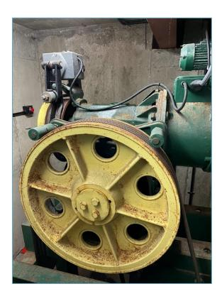
Escalators are not covered by LOLER (HMSO, 1998), but after a period out of service, the drive and steps chains may require lubrication.
