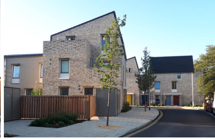
Goldsmith Street, Norwich City Council
