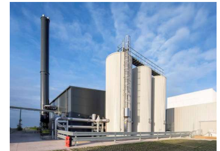
Shawfair Energy Centre, Midlothian Heat Network
