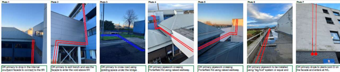
Photo 1: DH primary to drop in the internal courtyard facade to connect to the BR ventilation plant-room at L00. Photo 2: DH primary to exit trench and use the facade to enter the void above BR building. Photo 3: DH primary to cross road using existing space under the bridge. Distribution pipework to exit existing trench prior to building edge. Photo 4: DH primary pipework crossing Portersford Rd using raised walkway. Photo 5: DH primary pipework crossing Portersford Rd using raised walkway. Photo 6: DH primary pipework to be installed using "big foot" system or equal and approved. Photo 7: DH primary drops to plant-room D on the facade and enters at HL.
